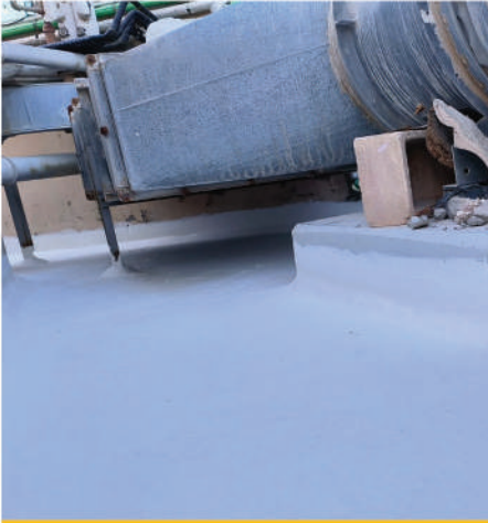
WATERPROOFING CLIENT : KEMPINSKI RESIDENCES
