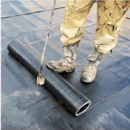
Bitumen Membrane Waterproofing
