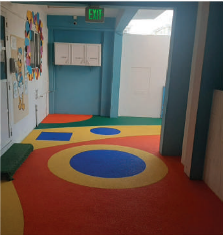
EPDM WORK CLIENT : DAFFODILS NURSERY
