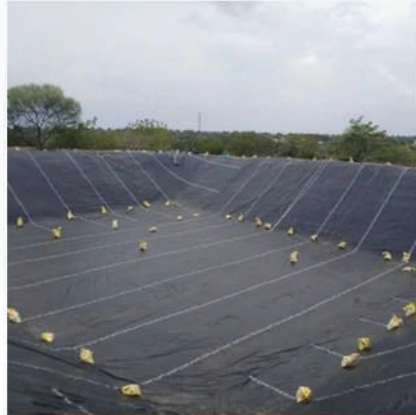
HDPE Membrane Waterproofing
