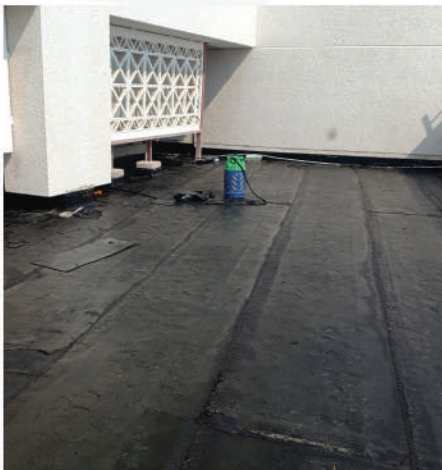
WATERPROOFING CLIENT : THE RITZ-CARLTON HOTEL
