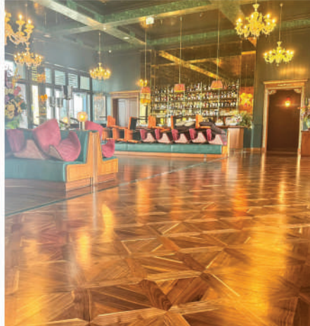
FLOOR POLISHING WORK CLIENT : CARBONE RESTAURANT
