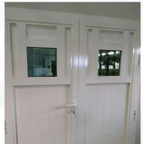
FITOUT WORK CLIENT : AL MANHAL WATER FACTORY
